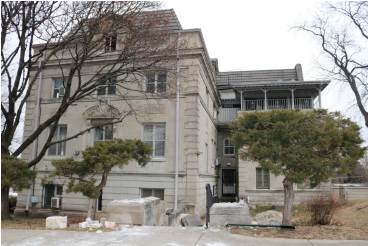
Directly south of Chancery Building, 12/19/2018
