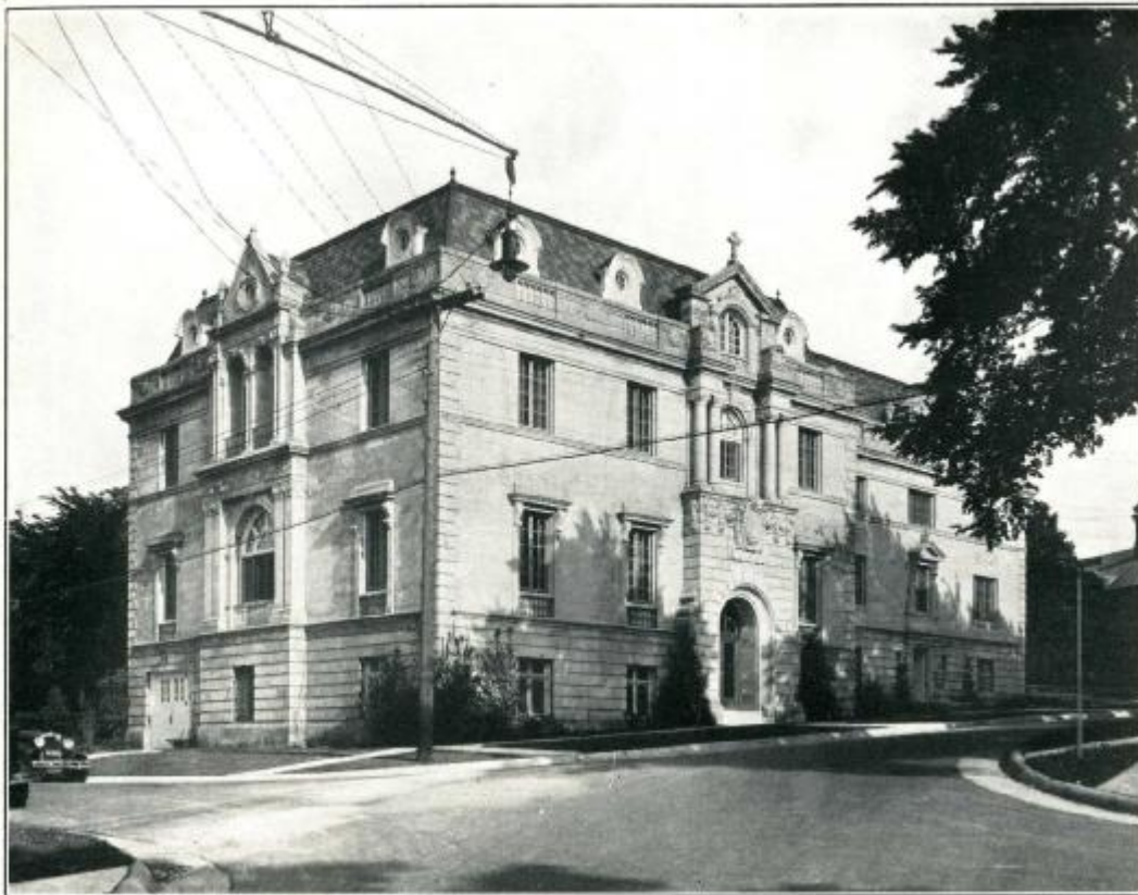
NORTH AND WEST FACADES
