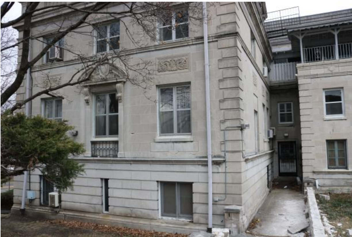
Directly south of Chancery Building, 12/19/2018
